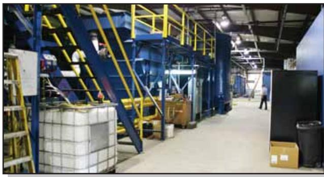
Raw wastewater from the well site is delivered to the Eureka facility by development companies where it is evaluated and tested prior to processing. Plant operators provide a preliminary analysis and assessment of the water for dissolved solids, barium, settled solids, mud and oil.
